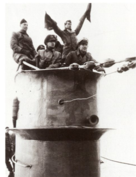
Right: U121, a small coastal boat of Type IIB. The signalman and the absence of lookouts suggest that this photograph was probably taken while entering or leaving port. A wire can be seen running from the radio intake connector to the stout jumping wires which served as aerial and attachment for safety harness when men worked on the upper deck. The other round object, lower down towards the right, is a fog horn.
